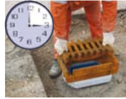
15. Min.: assembly of grating
