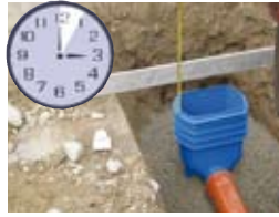
5. Min.: height adjustment
