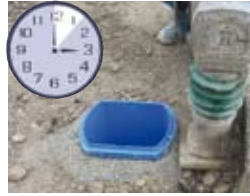
7. Min.: backfilling and compacting
