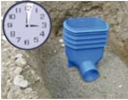
3. Min.: bedding in lean concrete mix
