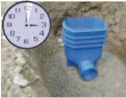
3. Min.: bedding in lean concrete mix
