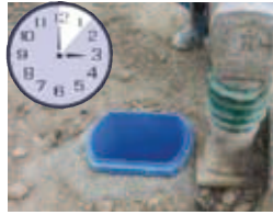
7. Min.: backfilling and compacting
