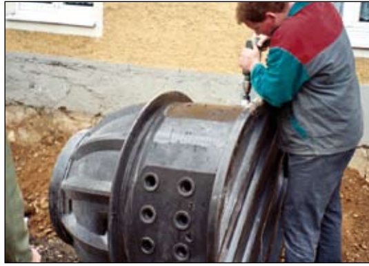
Pipe joint and seal installation on site
