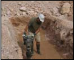
Prepare and compact the construction pit
