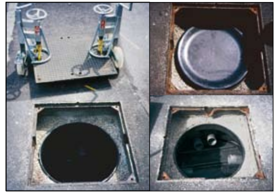
Watertight cover system with separate sealing and bearing function.
