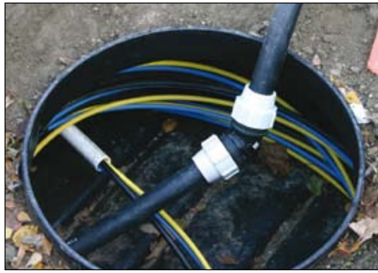
Placement of reserve cables in watertight ROMOLD PE chambers.
