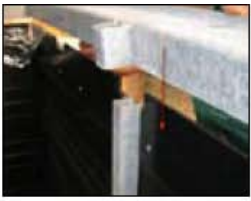
Connect the vertical profiles to the chamber cover frame using the plug-in system.
