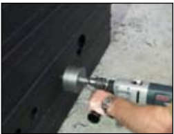
Insertion openings made by the customer
